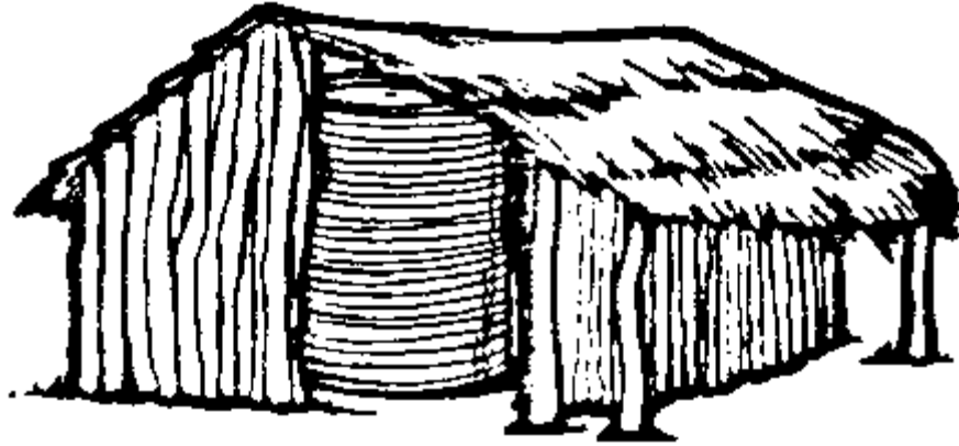
Fig. 58: These silos were imported as a development project. It was soon found that farmers could not afford them, that they heated and cooled rapidly, causing condensation and that they rusted through in three or four years.
