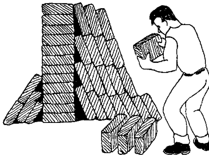
Figure 46. Adobe block is stacked after a month of curing.
